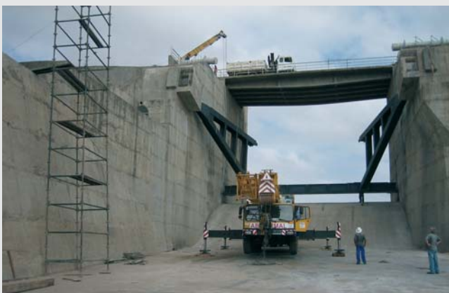
Montage Segmentschütz - Installation Radial Gates
