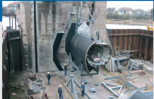
Einheben Walze – Placing of Drum Gate
