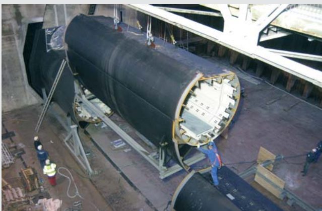
Montage Walze – Installation Drum Gate
