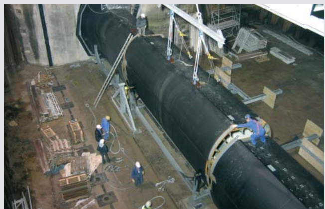
Montage Walze – Installation Drum Gate
