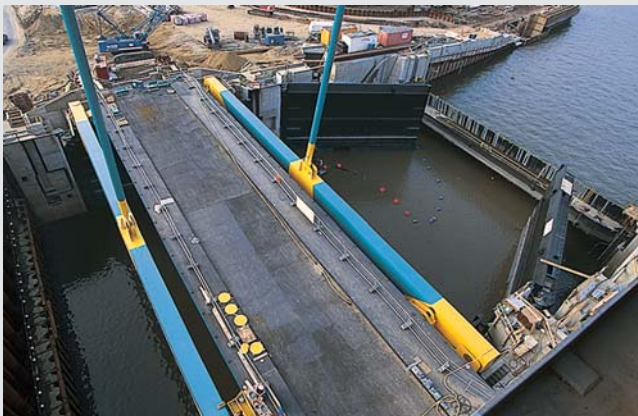
Montage Klappbrücke - Installation Bascule Bridge
