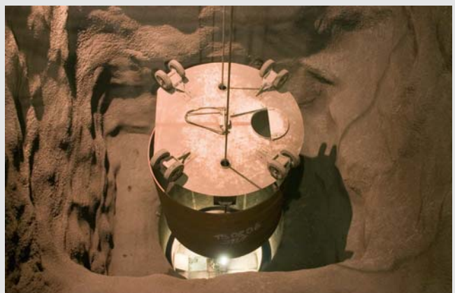
Absenken Rohre - Lowering of Cans
