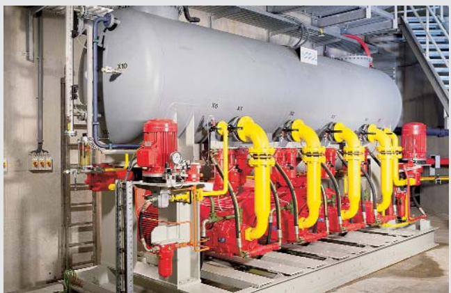
Hydraulikaggregat - Hydraulic Power Units
